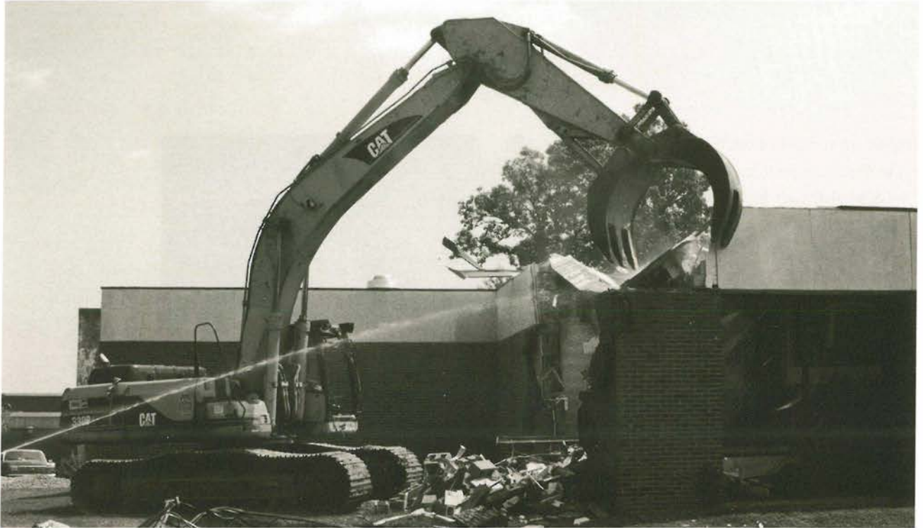
The demolition of Café North begins.
